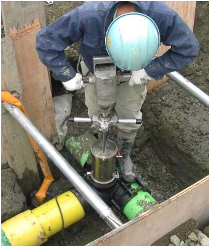
Figure 9 : The sight of work ( Boring hole with the specialized hot tapping tool )
