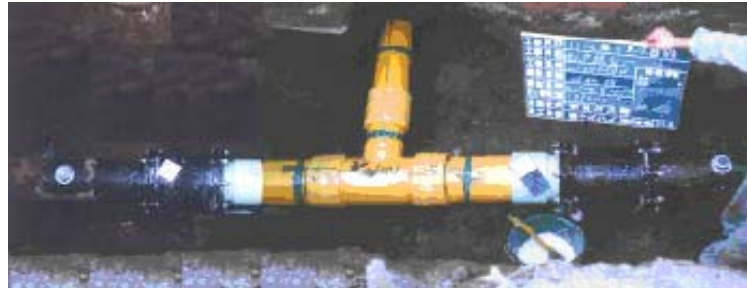
Figure 7 : Picture of the traditional hot branching technique
