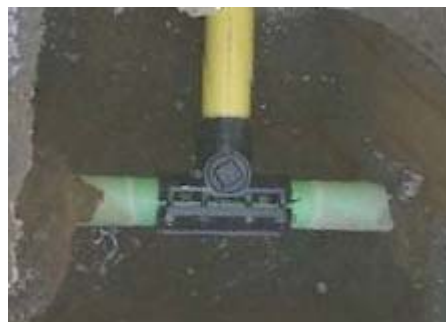
Figure 8 : Picture of the new hot branching technique
